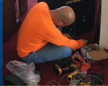
Deferred Maintenance of Church Buildings
